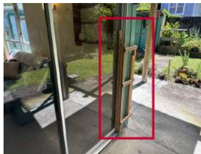
#37: temporary securing of fixed door sash
