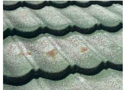
#127: rust deterioration
