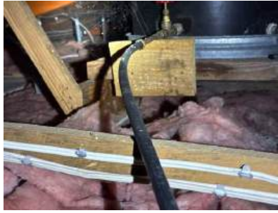
#204: black pipe in roof space
