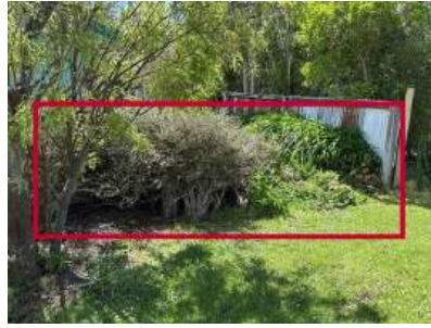
#250: wire fence has fallen down at front of property
