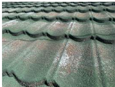
#132: coating deterioration
