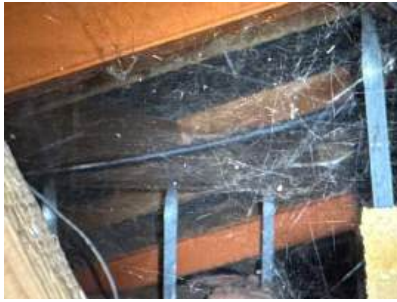
#206: black pipe in roof space
