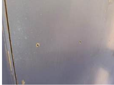
#72: nail holes exposed in liners
