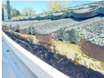
#126: rust deterioration
