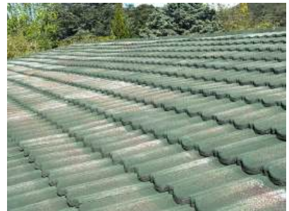
#130: coating deterioration
