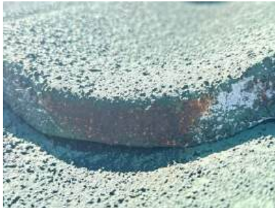
#125: rust deterioration
